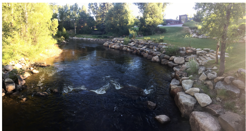
Recreation and bank stabilization structures above town.
