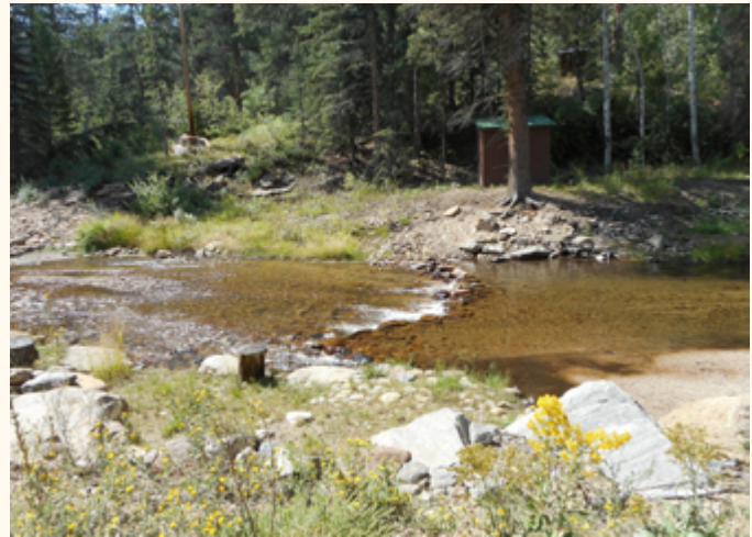
Grade control structures can control river form Photo by Kim Lennberg, Alba Watershed Consulting
