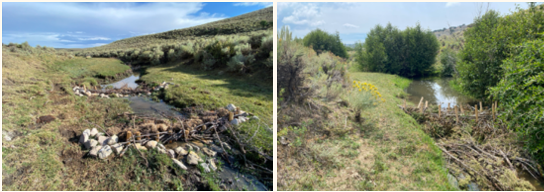
Beaver dam analogs cause pooling, reducing stream power and encouraging deposition Photos courtesy of Joe Leonhard, The Nature Conservancy
