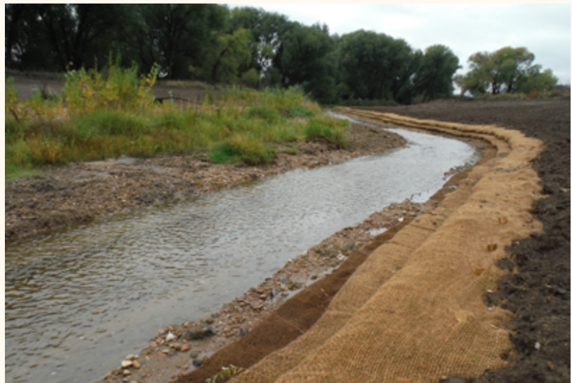
Soil lifts during construction Photo by Kim Lennberg, Alba Watershed Consulting
