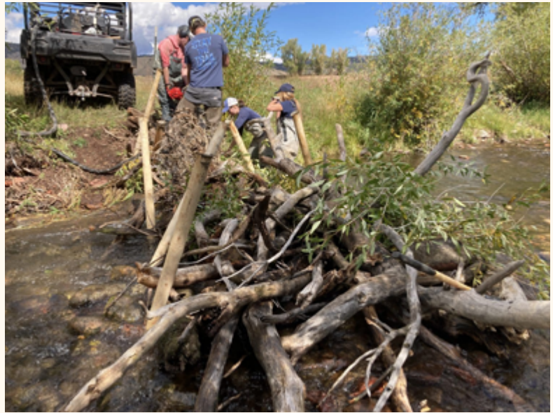
Surface-placed large wood structure intended to create more complex flow and scour patterns, as well as provide cover and structure for fish Photo courtesy of Eagle County Open Space
