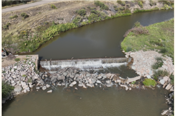
The pool below the dam, on the right side of the picture, is designed to help trout jump past the diversion. This is a barrier, however, to species that cannot jump such as suckers and sculpin. Photo by Roddy Beall, Zenobia Consultants
