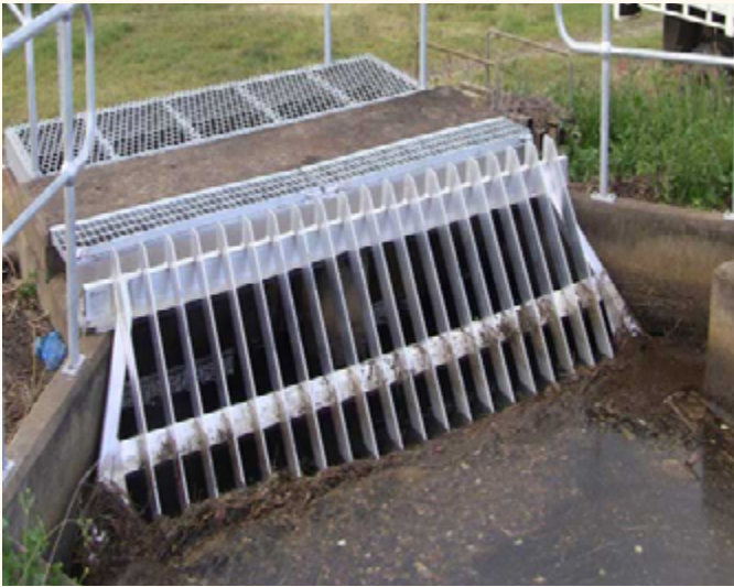
Adding a wood debris rack protects the headgate so more wood can remain in the river | Photo By RK Trading Company
