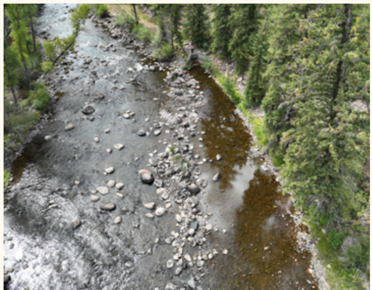
A boulder diversion structure allows fish passage | Photo by Roddy Beall, Zenobia Consultants
