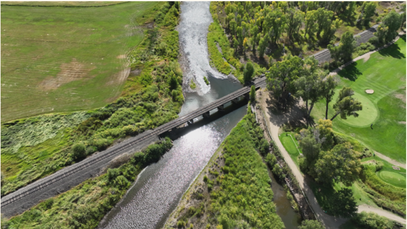
A railroad bridge causes unnatural river dynamics, leading to an odd angle and erosion problems Photo by Roddy Beall, Zenobia Consultants
