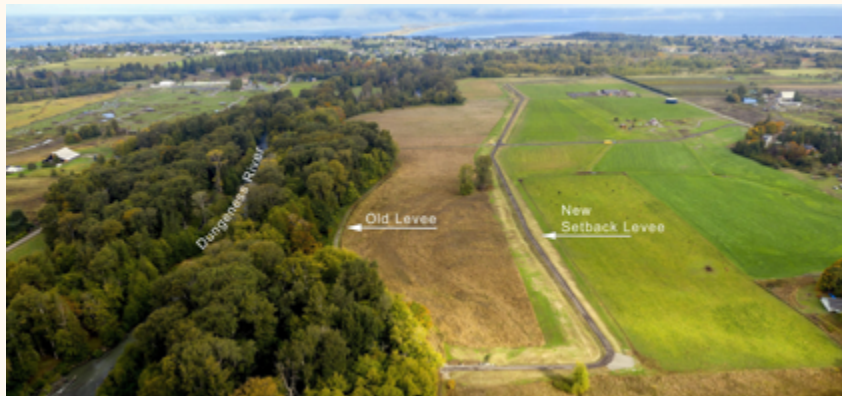
A setback berm in Washington replaces an old levee located close to the river | Photo by Tiffany Royal, Jamestown S'Klallam Tribe
