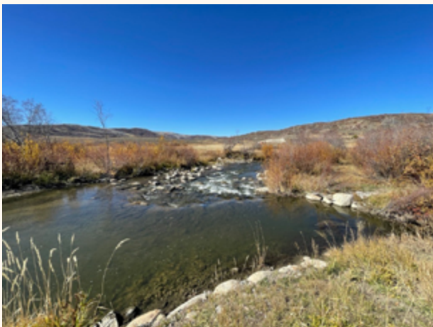
A diversion structure with an ecological rock ramp feature that allows for fish and sediment passage Photos and Project by Flywater, Inc.
