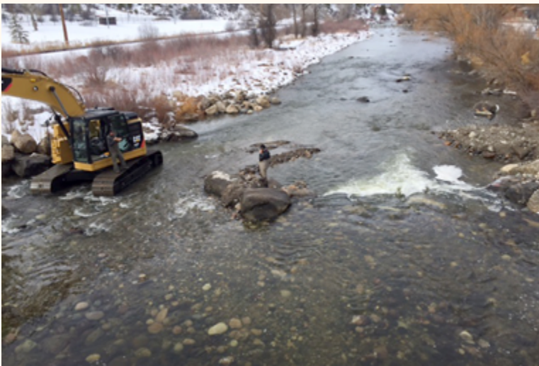
Excavators build a boulder structure where wood structures are not possible | Photo by Peter Van De Carr
