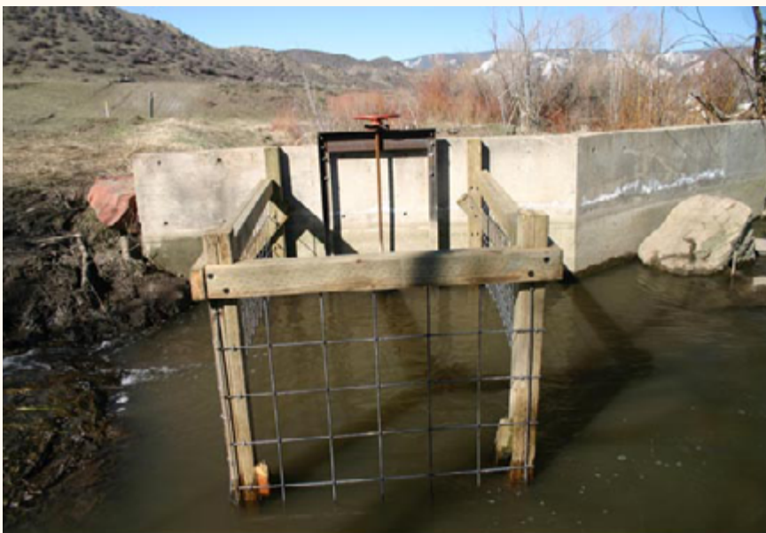
A flow device on an irrigation headwall protects the ditch without the need to remove beavers | Photo courtesy of Skip Lisle, Beaver Deceivers International
