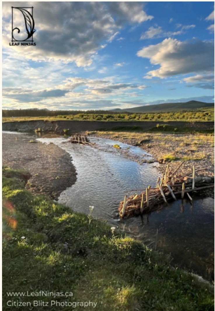
Post-assisted log structures redirect stream flow to reduce erosion and increase deposition where desired | Photo by Leaf Ninjas
