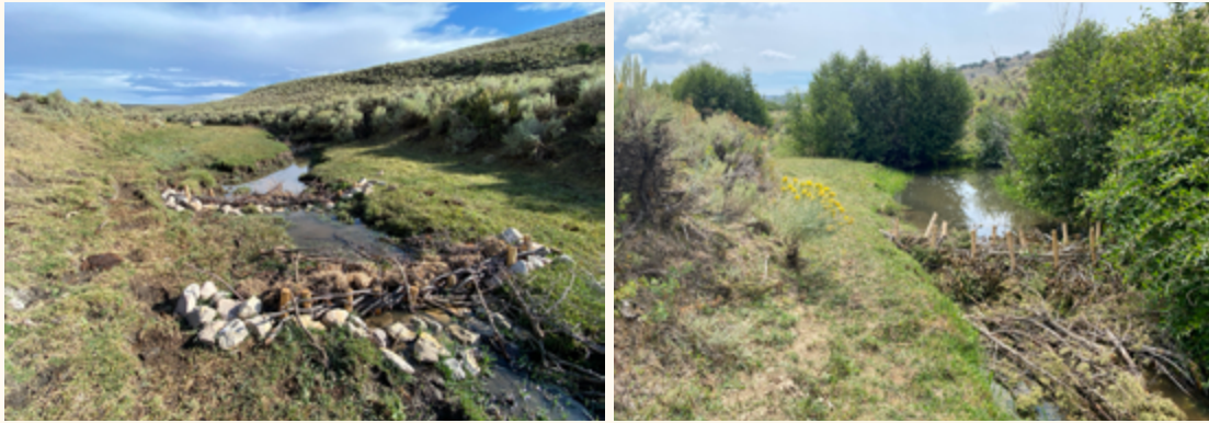
Beaver dam analogs cause pooling, reducing stream power and encouraging deposition Photos courtesy of Joe Leonhard, The Nature Conservancy
