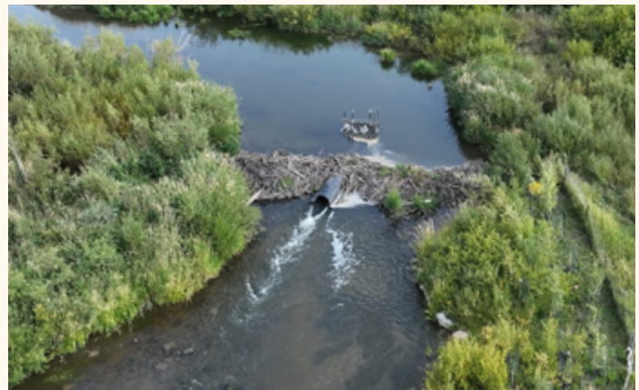
A pond leveler maintains the pond level at a certain height Photo by Roddy Beall, Zenobia Consultants
