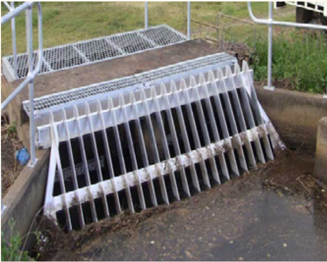
Adding a wood debris rack protects the headgate so more wood can remain in the river | Photo By RK Trading Company
