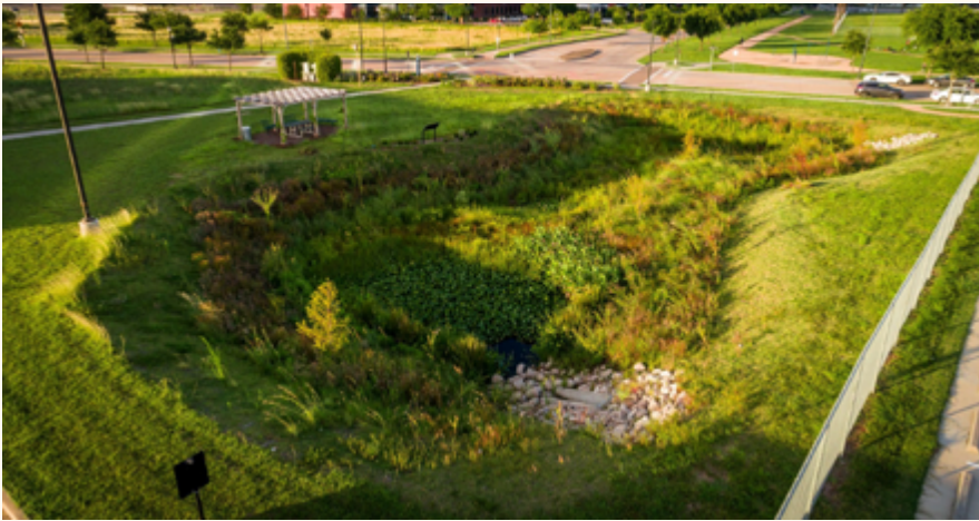
For urban runoff or irrigation return flows, an infiltration pond filters water through sedimentation and wetland plants | Photo courtesy of Bryan Malloch
