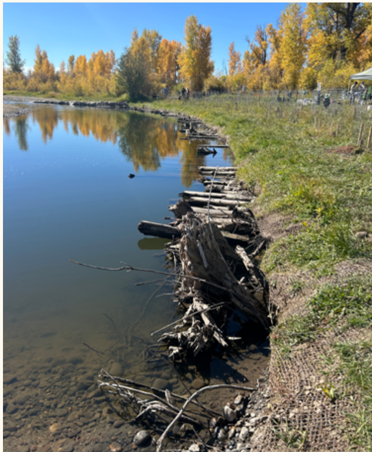
Toe wood and bankfull bench at Chuck Lewis State Wildlife Area Photo by Ben Beall, Zenobia Consultants
